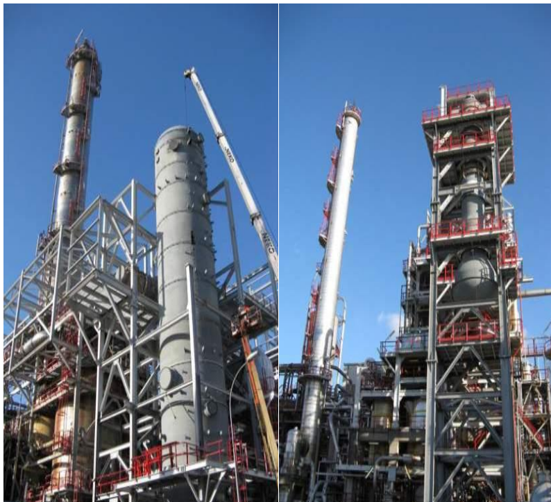
BP Geel PTA Project – 12 pics; Belgium – Technip; SB265 Gr.1/SA516 Gr.70N
