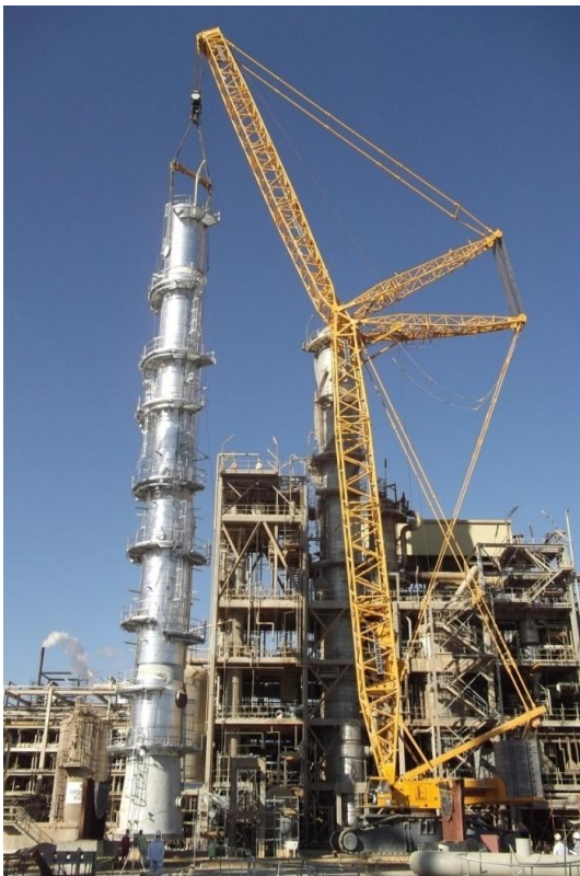
SABIC PTA Project - Saudi Arabia; Titanium clad, SS316L, S32205, 20 pics
