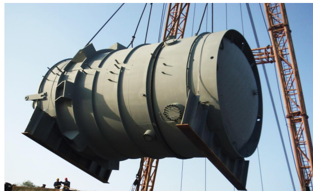
Crystallizer DN7100mm;TA1/Q235A
